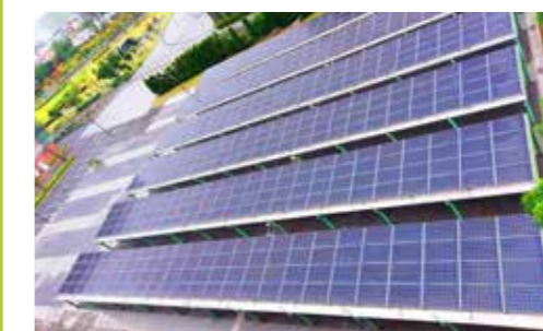
▲ Taoyuan-Solar Power Generation System
