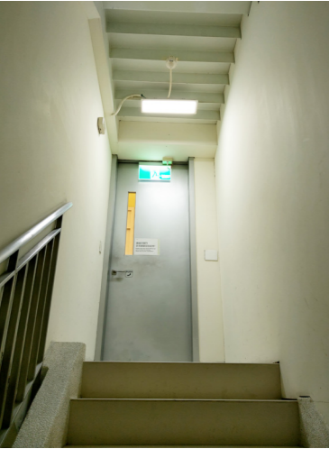
Infrared switch of safety ladder lighting
