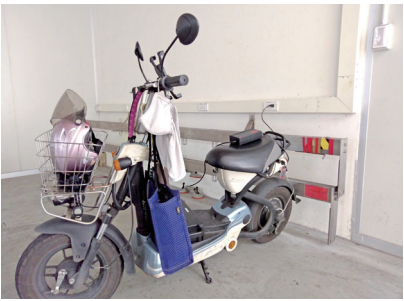
Power charging sockets for electric vehicles
