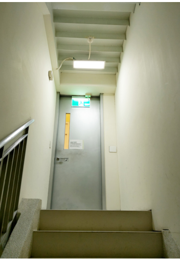
Infrared switch of safety ladder lighting
